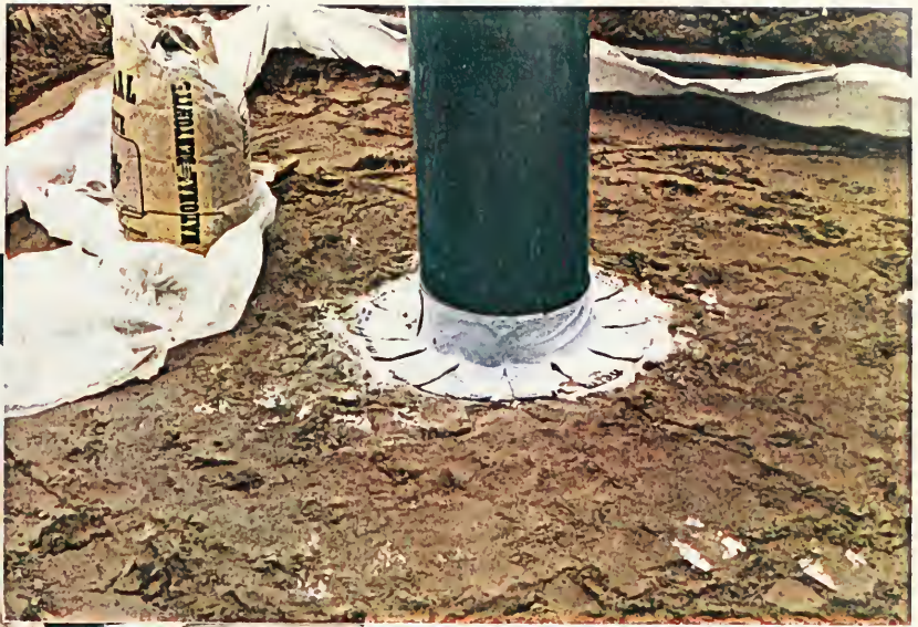
A 16: BENTONITE PLACED BELOW THE TWO MEL-ROL MEMBRANE LAYERS SHOWN INSTALLED
